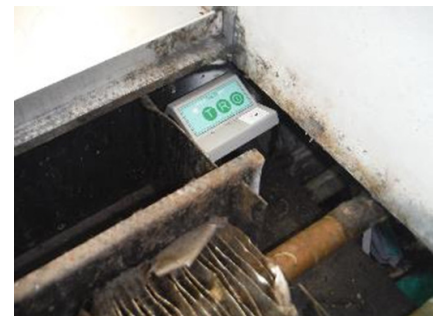
Fig 3: GT sensor mounted on bracket
